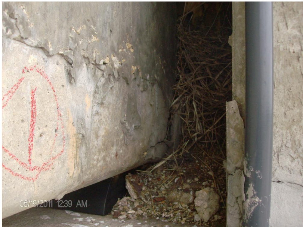
Photo 20: Excessive debris between Beam 1 and screen wall at the South Abutment
