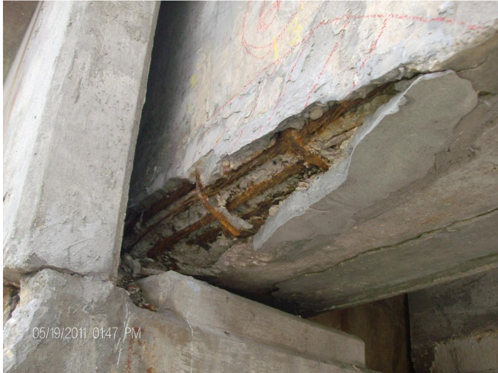
Photo 11: Beam 6 Spalling & Delamination at the South Abutment
