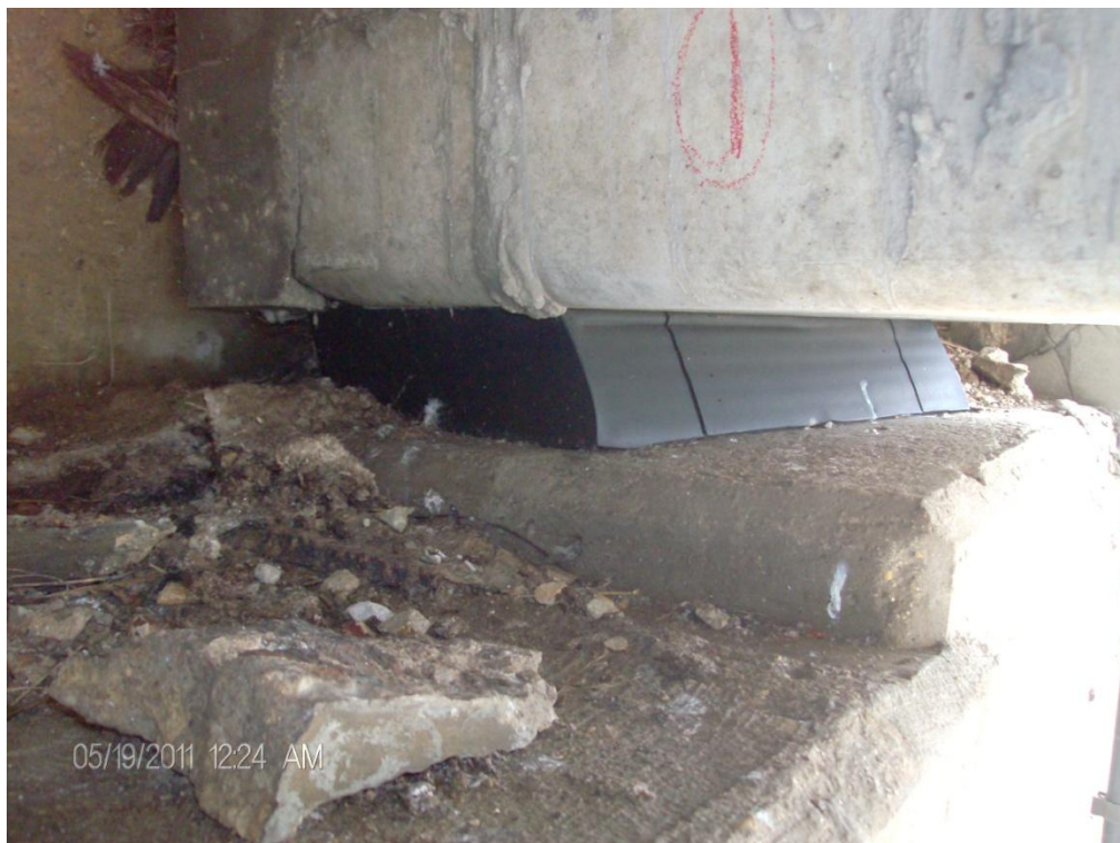
Photo 12: Slight lift-off of Beam 1 Bearing corner at South Abutment
