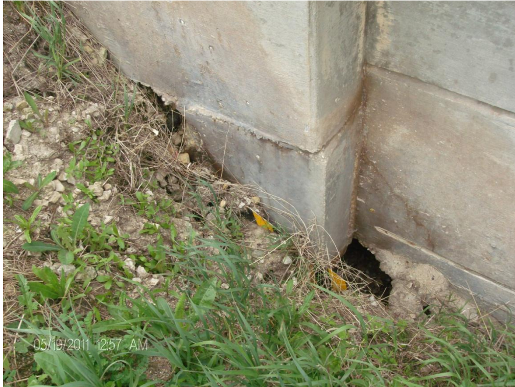
Photo 23: 18' long x 3' wide x 3' deep washout at the Southeast Curtain Wall
