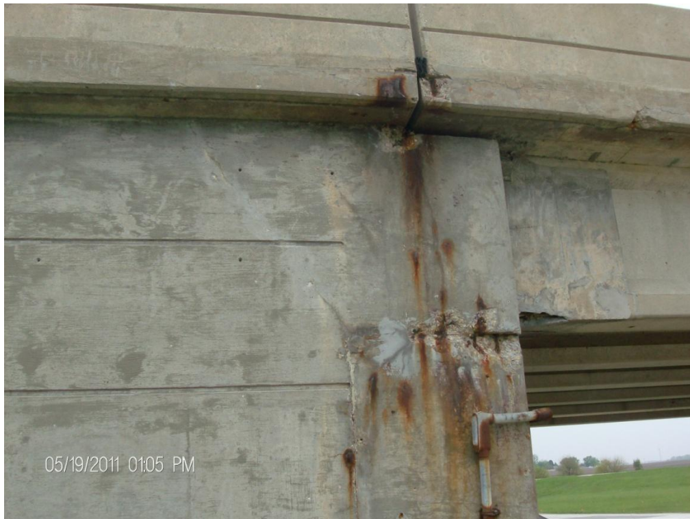
Photo 24: Spalling on Southeast Curtain Wall
