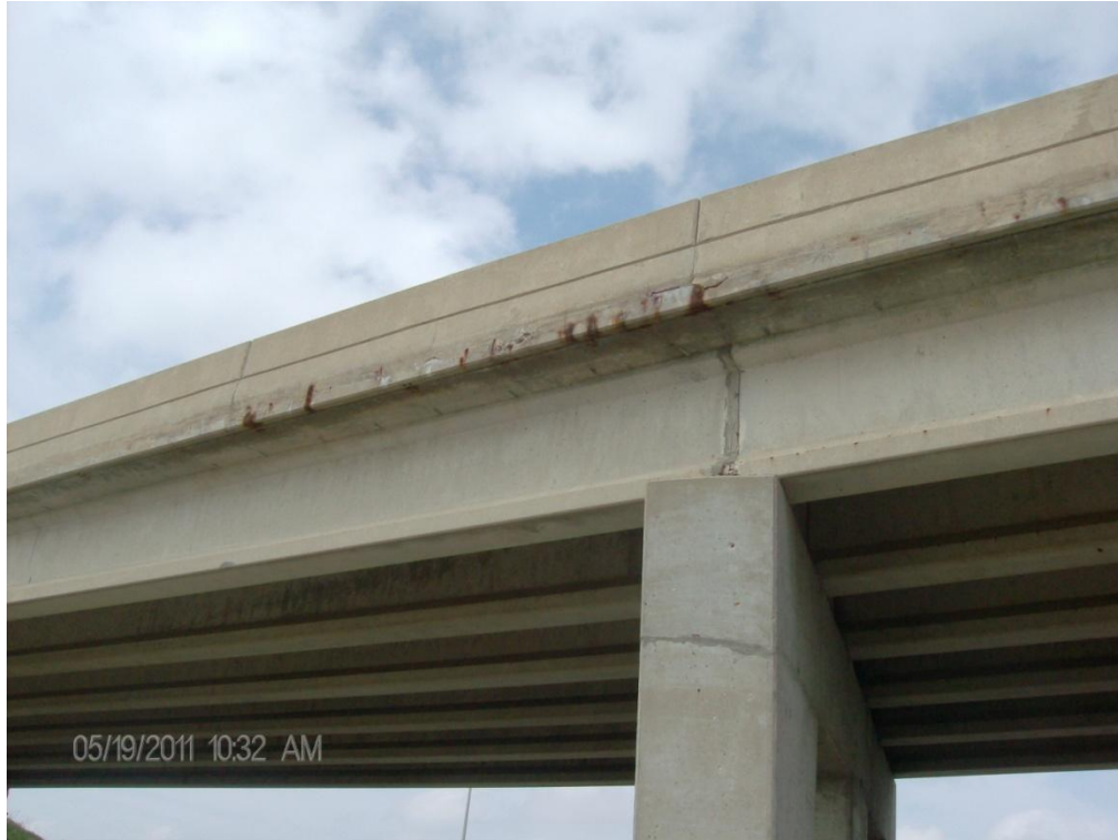
Photo 5: Spalling & Delaminations along the bottom 1' of East Parapet, about 20' long
