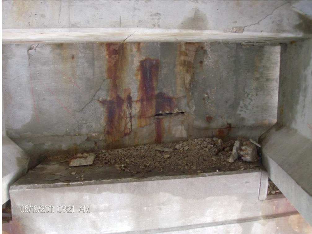
Photo 19: Debris build-up between Beams 3 and 4 at the North Abutment
