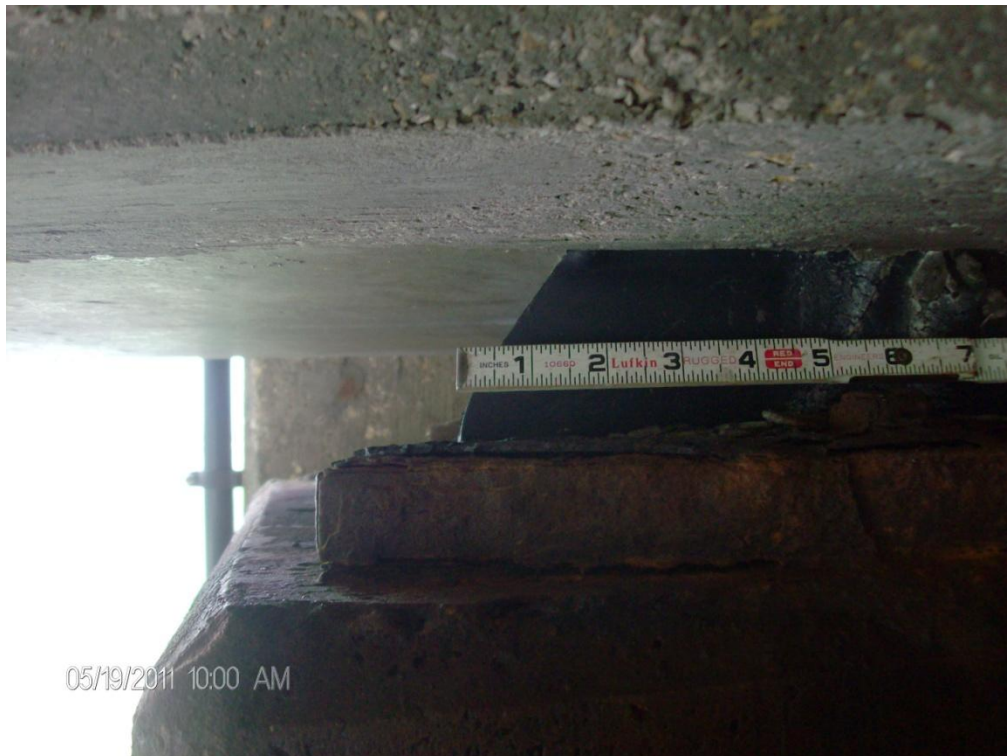
Photo 14: Beam 1 North Abutment bearing expanded about 1½" in 65° weather
