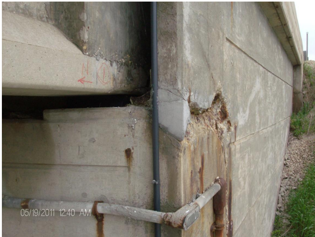
Photo 22: Spalling and deterioration at the Southwest Curtain Wall and Screen Wall
