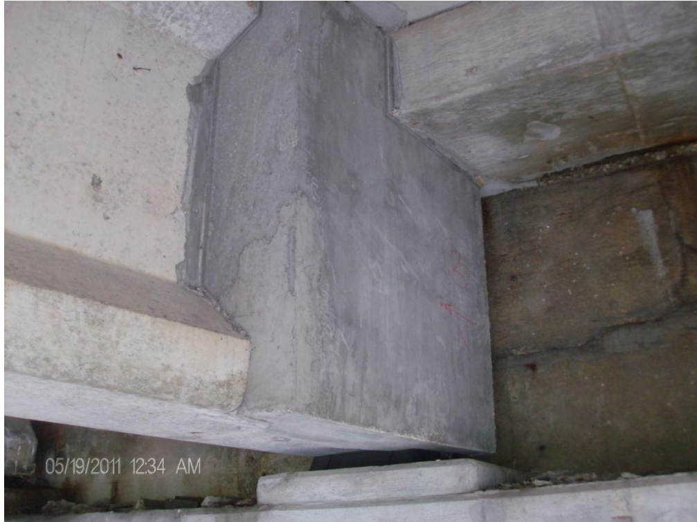
Photo 9: Concrete End Encasement at South Abutment, Beam 2
