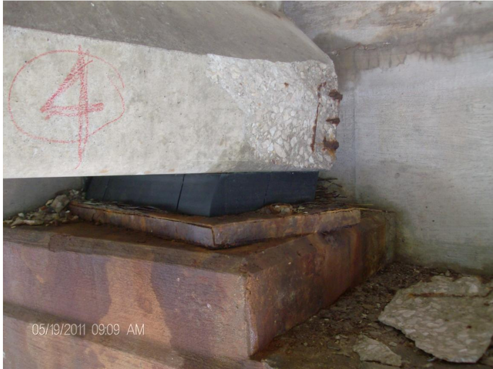
Photo 13: Heavy rusting & flaking at Beam 4 Bearing, North Abutment
