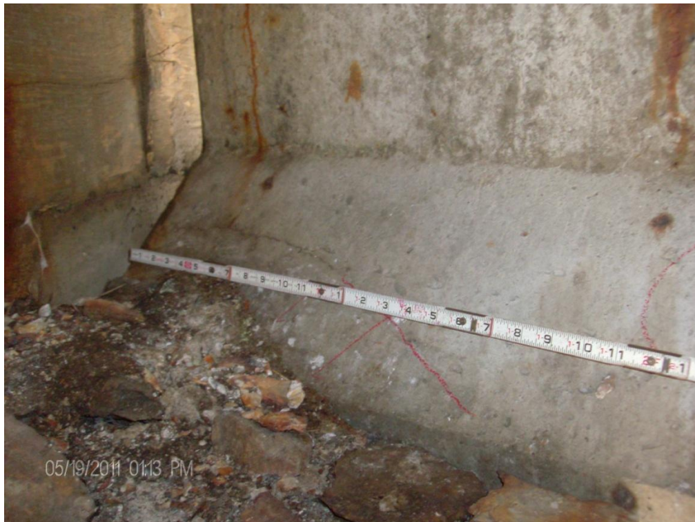
Photo 10: Beam 3 bottom flange delamination at the South Abutment
