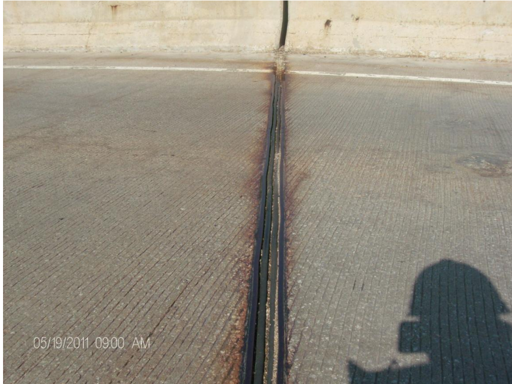
Photo 7: SB Expansion Joint at South Abutment
